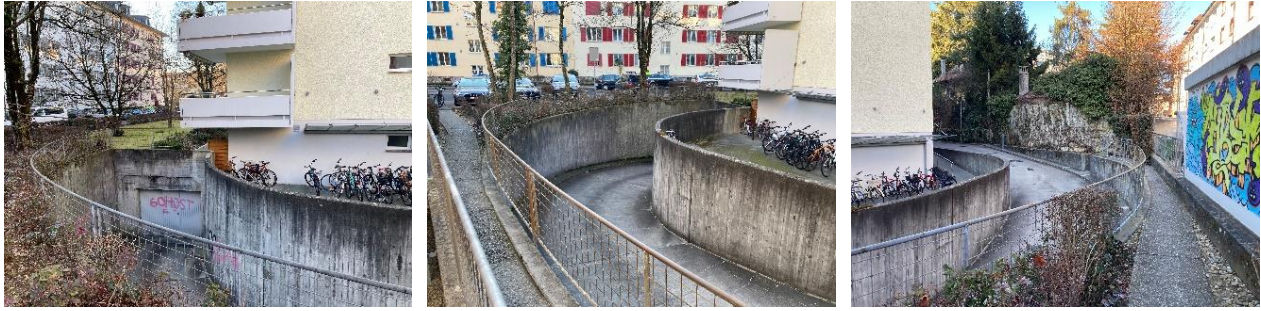
Figure 43: Three pictures showing hazard area #2 (own images taken on 13.01.2022)
